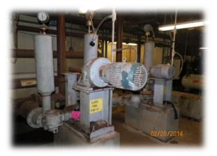
The current pumps are original to the building in 1980. They have been in constant use since then. They have been rebuilt several times but they are finally to the point of replacement.
