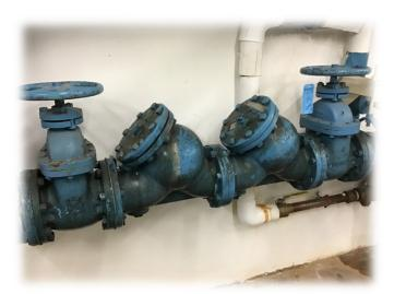
The facility has 9 back flow preventers thru out the plant, which must be inspected annually to insure that they are operating properly. The function is to prevent Non-Potable water from getting into the drinking supply. The facility currently has two that need to be replaced and another two that need to be repaired.
